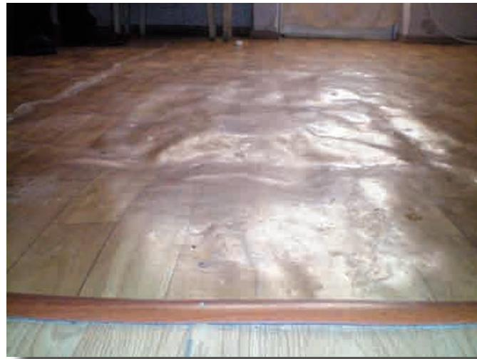
The inspection of the dormitory on site proved that the implementing entity has fulfilled somewhat quality works, although some quality violations were also detected. In particular, the kitchens lack a cement floor and oilcloth is just spread on rough floors.
